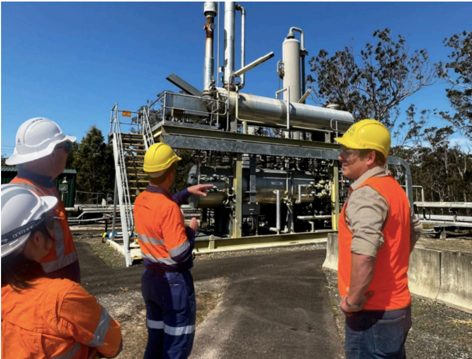
Underwood inspecting the offline RPGP with representatives of AGL and InGauge Energy.
