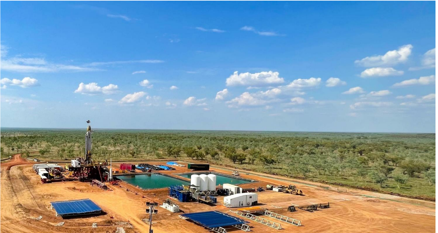
Silver City Drilling Rig 40 at the Carpentaria-2H well pad
