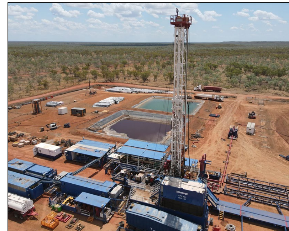
SLB 185 Rig drilling Carpentaria-3H in EP187
