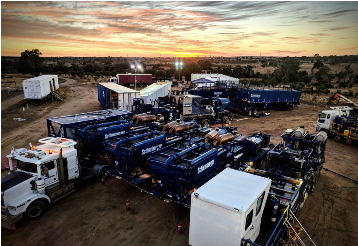
Illustrative example of hydraulic fracture stimulation equipment (Note: image is not from the Empire Carpentaria-1 location)
